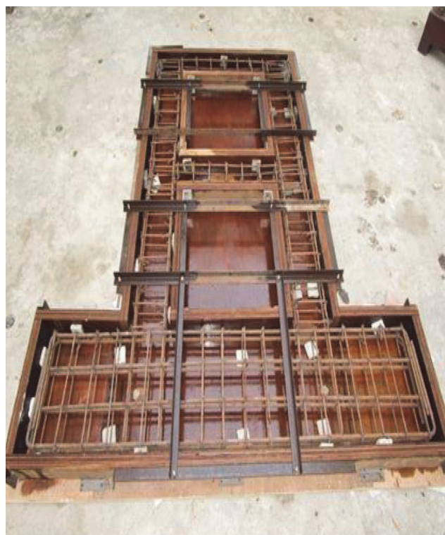
Figure 4. Mold with rebar arrangement
